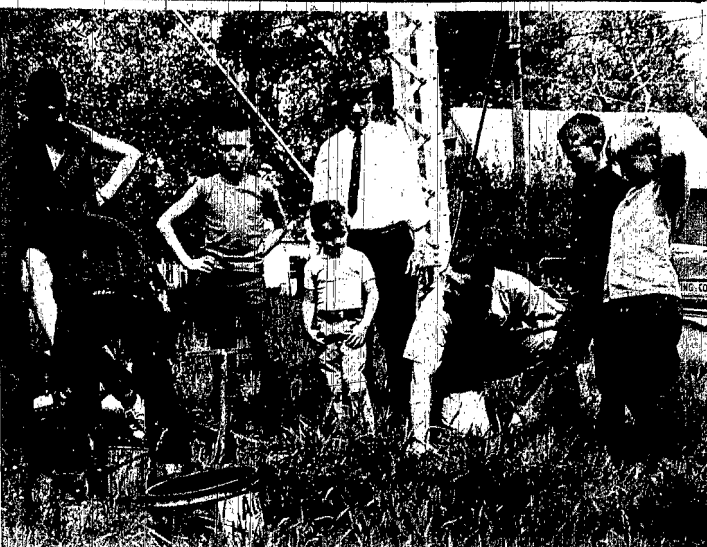
A BIG CREW was on hand Thursday to "help" repair the Concord water tower. Shown beneath the tower are Richard Jones (back to camera) and left to right, Steve Martindale, Alan Nobbe, Scott Nelson, Jerry Martindale, Mayor Bob Sherry, Randy Rees and Mark Martindale.
