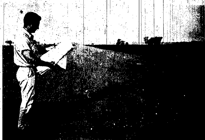
STRETCHING AWAY for 2,800 feet is the new runway for the Wayne Municipal Airport. The base is being put down now in prep for the surfacing. Joe Chamberlain, who is with Consolidated Engineers, Omaha, is shown checking plans Wednesday in the early morning hours.
